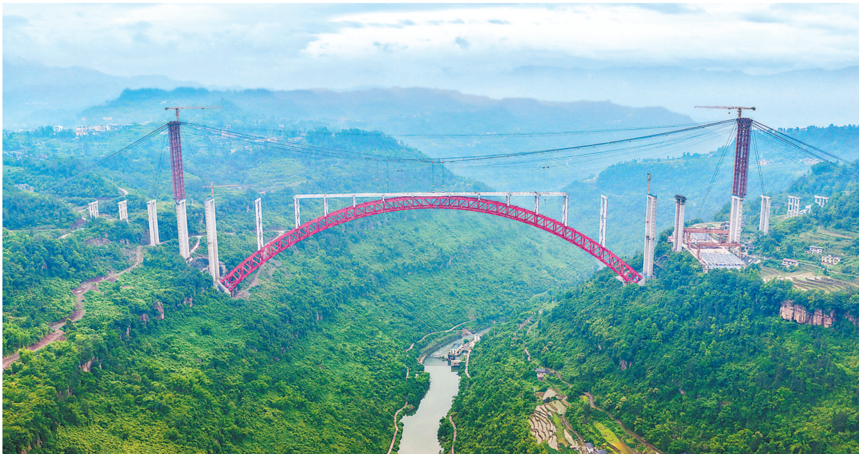
The Fenglai Daxi River Grand Bridge under construction in southwest China's Chongqing. (PHOTO: XINHUA)
