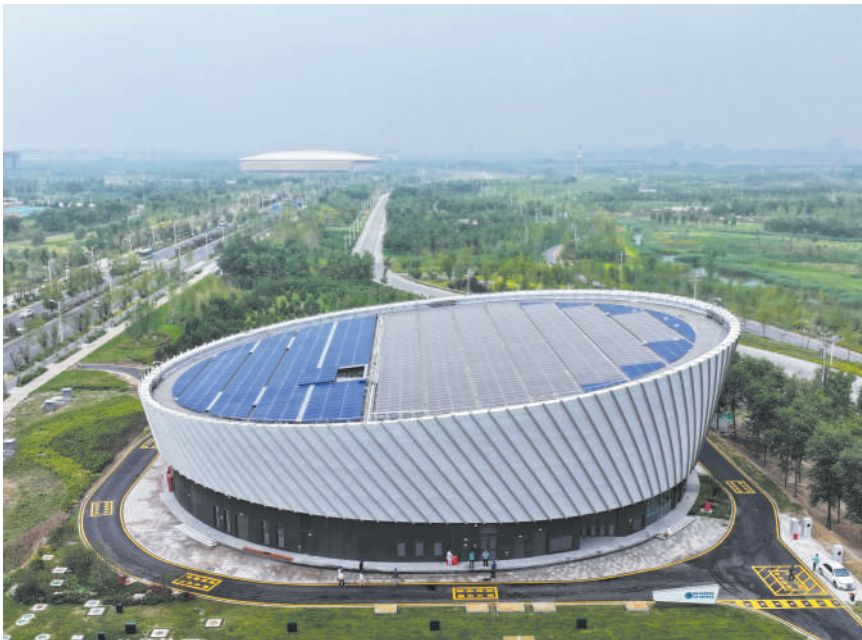
The Fuxing 220-kilovolt substation, Xiong'an New Area's first full-lifecycle near-zero carbon facility in Hebei province. (PHOTO: XINHUA)
