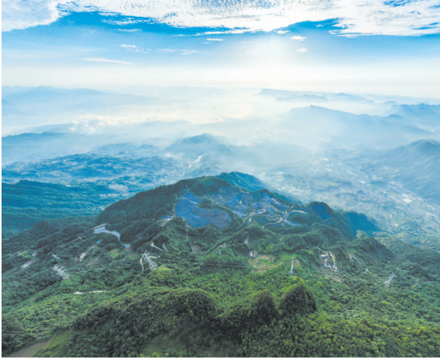
A photovoltaic power plant in Sixi village, Yichang city, central China's Hubei province. (PHOTO: VCG)
