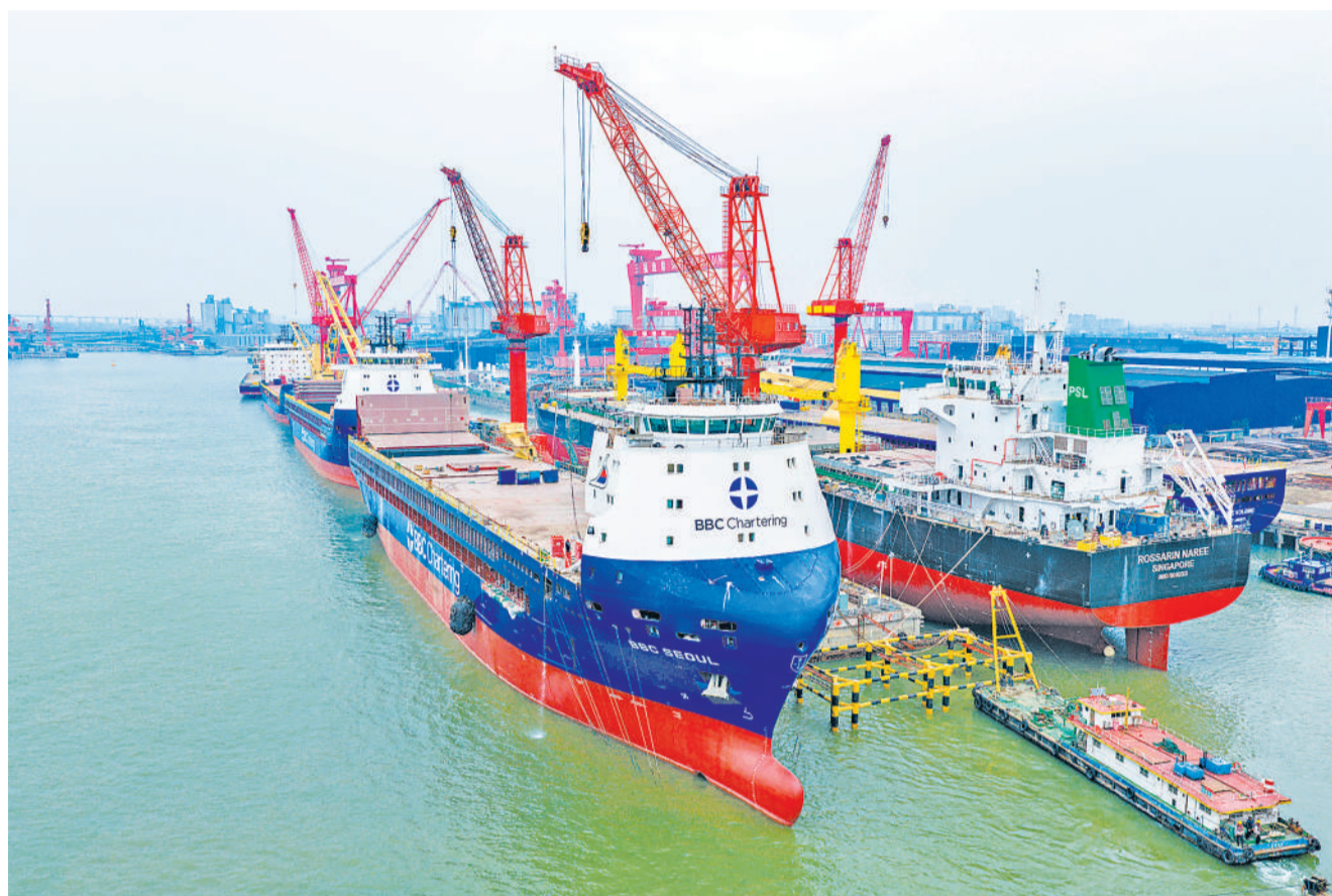
Several large ships are under construction in Taizhou city, Jiangsu province on February 2. Latest data from China's Ministry of Industry and Information Technology show that the country maintained a leading position in the global market share for shipbuilding for 16 consecutive years. (PHOTO: XINHUA)
