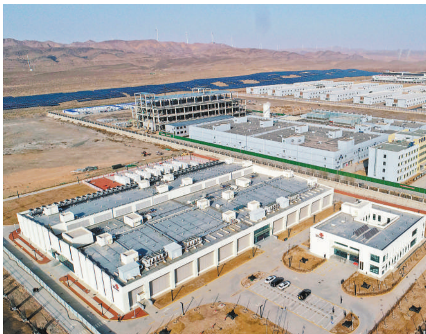
The photo shows a data center in Zhongwei city, Ningxia Hui autonomous region. (PHOTO: XINHUA)
