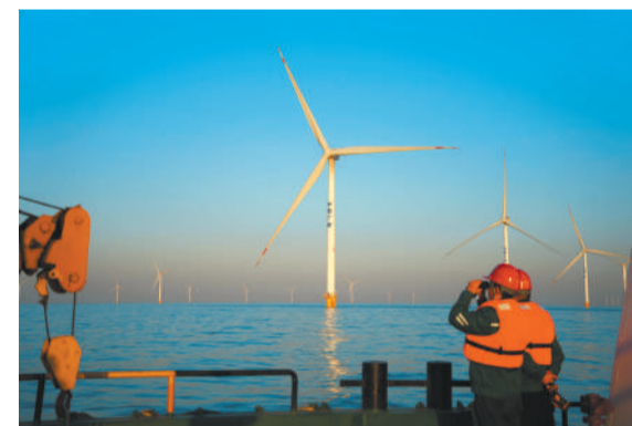
The photo taken on January 7, 2025, shows the offshore wind power project area of Laidou city, Shandong province. (PHOTO: XINHUA)
