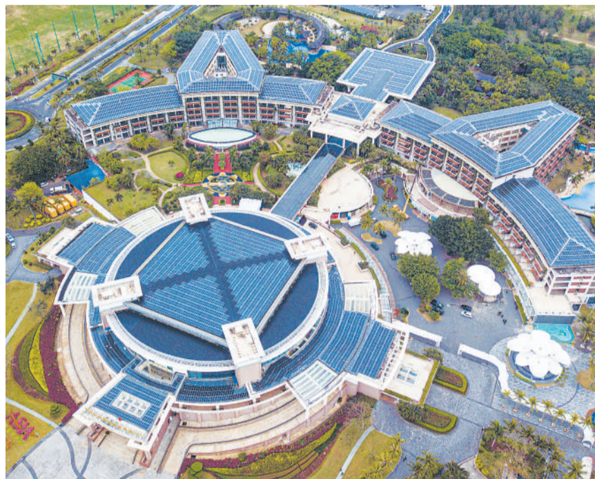
The photovoltaic devices on the roof of the Boao Forum for Asia (BFA) International Conference Center and a BFA hotel in the Boao zero-carbon demonstration zone in Boao, south China's Hainan province. (PHOTO: XINHUA)
