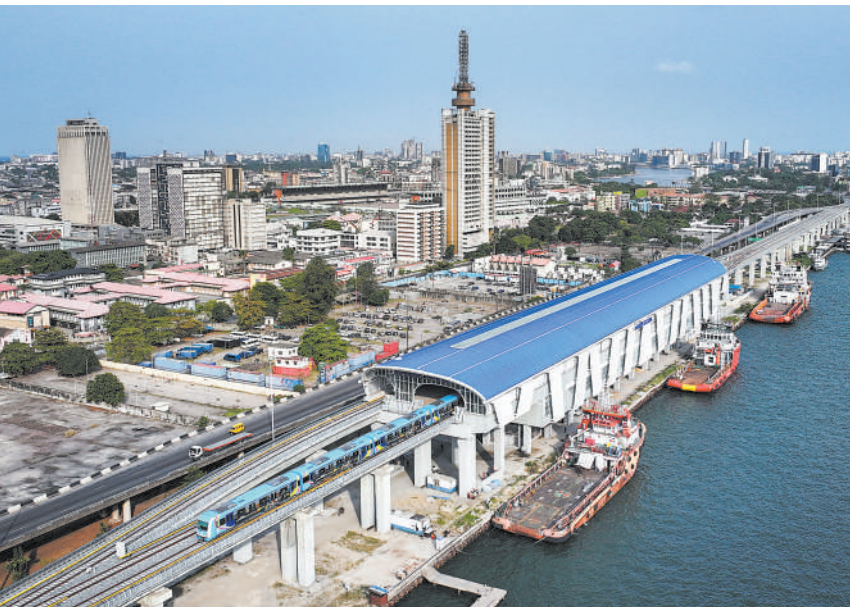
A train of the Lagos Rail Mass Transit (LRMT) Blue Line pulling in the Marina Station in Lagos, Nigeria. (PHOTO: XINHUA)
