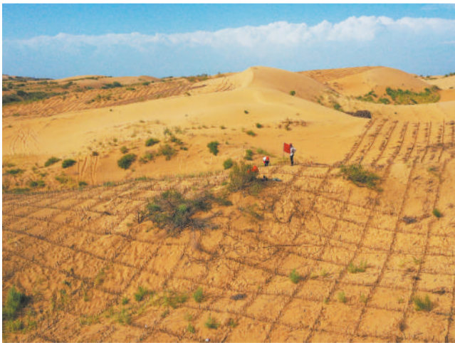
Workers set up straw checkerboards to prevent wind and fix sand in the Kubuqi Desert, China's seventh-largest desert, nestled in the northern part of the Ordos Plateau in Inner Mongolia. (PHOTO: XINHUA)
