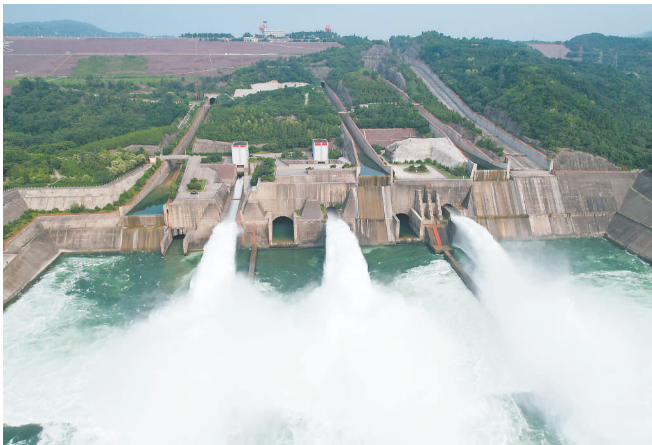
Aerial photo shows a water and sediment regulating operation carried out at Xiaolangdi Reservoir on the Yellow River in Jiyuan, Henan province, central China. (PHOTO: XINHUA)
