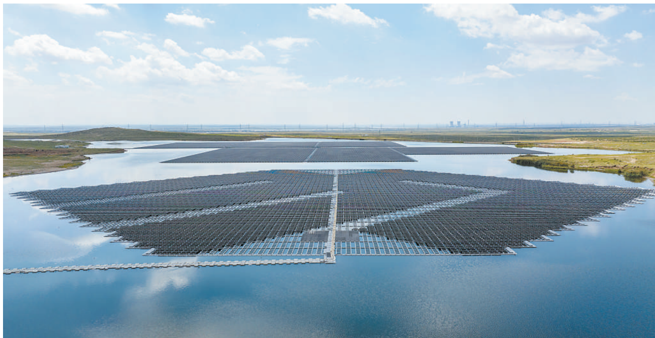
A floating distributed photovoltaic power generation project in Lingwu city, Ningxia Hui autonomous region. (PHOTO: XINHUA)
