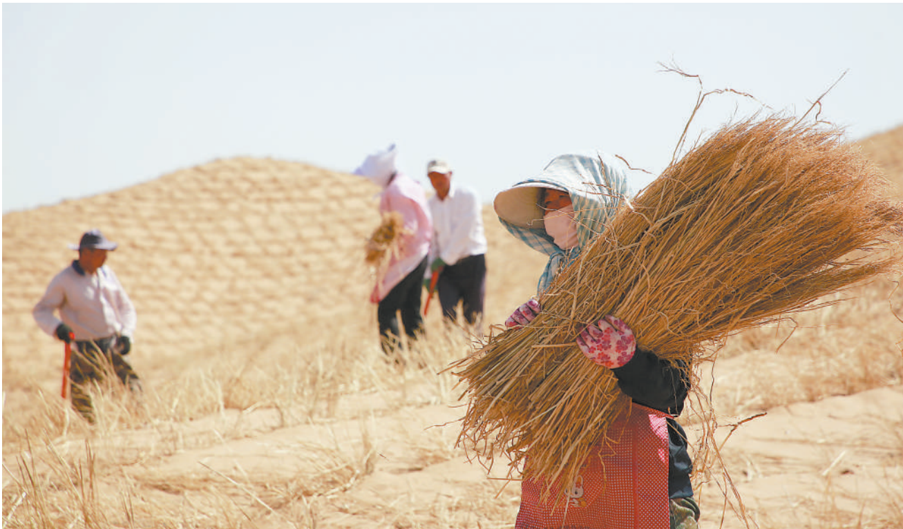
Workers make straw checkerboards in the Tengger Desert in Zhongwei, northwestern China's Ningxia Hui autonomous region, on May 9, 2024. (PHOTO: VCG)
