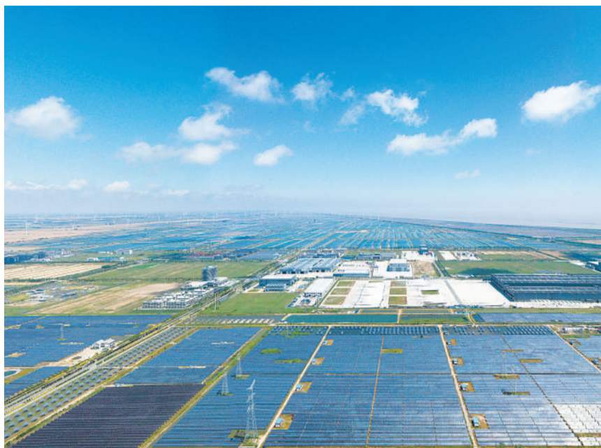
An aerial view of a low (zero) carbon-dioxide emission industrial park in Sheyang, Yancheng, east China's Jiangsu province. (PHOTO: XINHUA)
