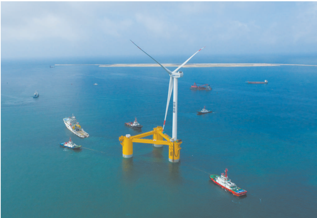
Equipped with 6.2 megawatt typhoon-resistant wind power generating units, China's first deep-sea floating wind power equipment "Fuyao" was towed in Maoming, south China's Guangdong province on May 29. (PHOTO: XINHUA)
