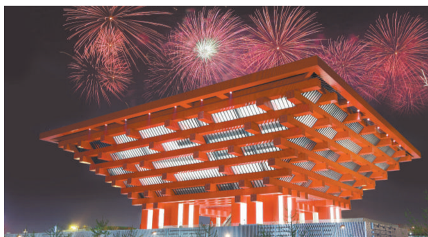
China National Pavilion of World Expo 2010 Shanghai, typical mortise and tenon structure "dougong (corbel bracket)." (PHOTO: VCG)
