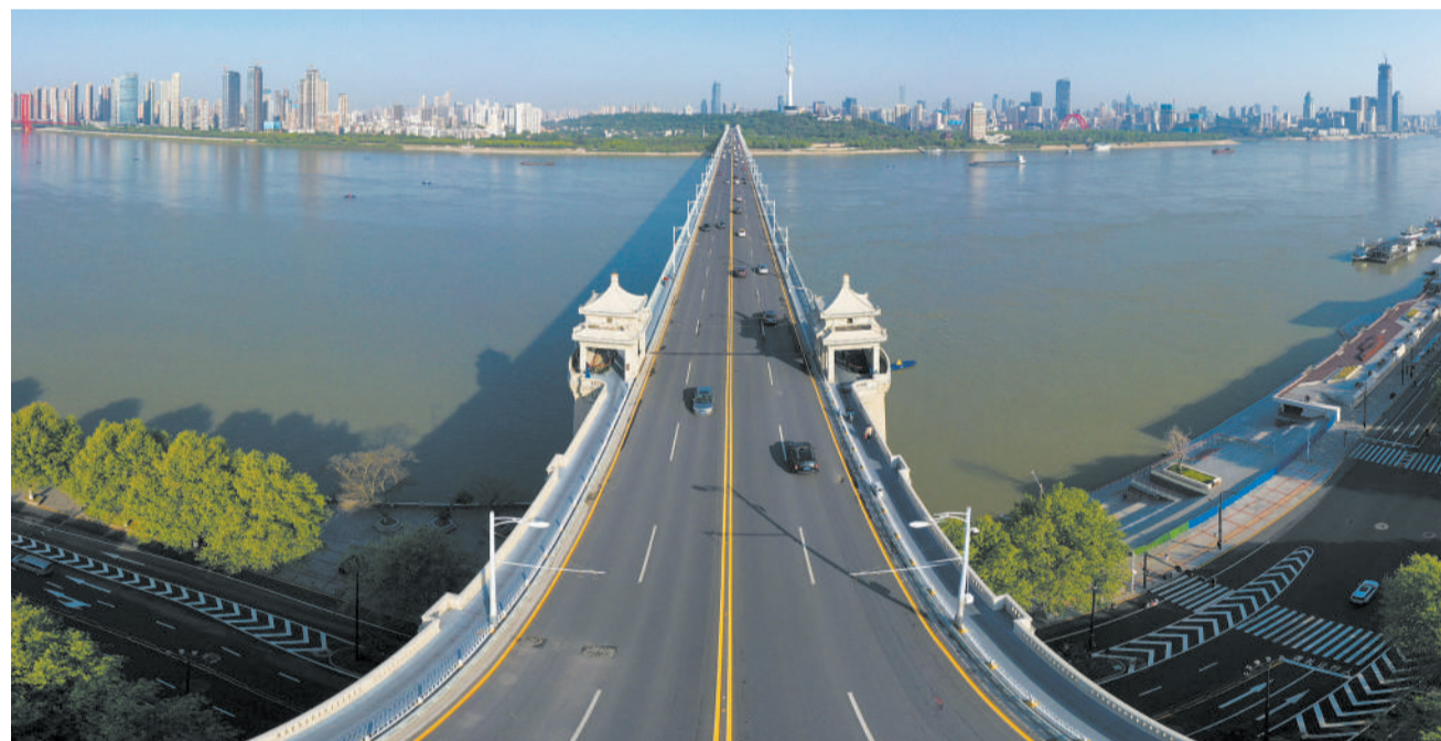
Wuhan Yangtze River Bridge in China's Hubei is the first major bridge across the country's busiest and longest waterway of Yangtze. (PHOTO: XINHUA)
