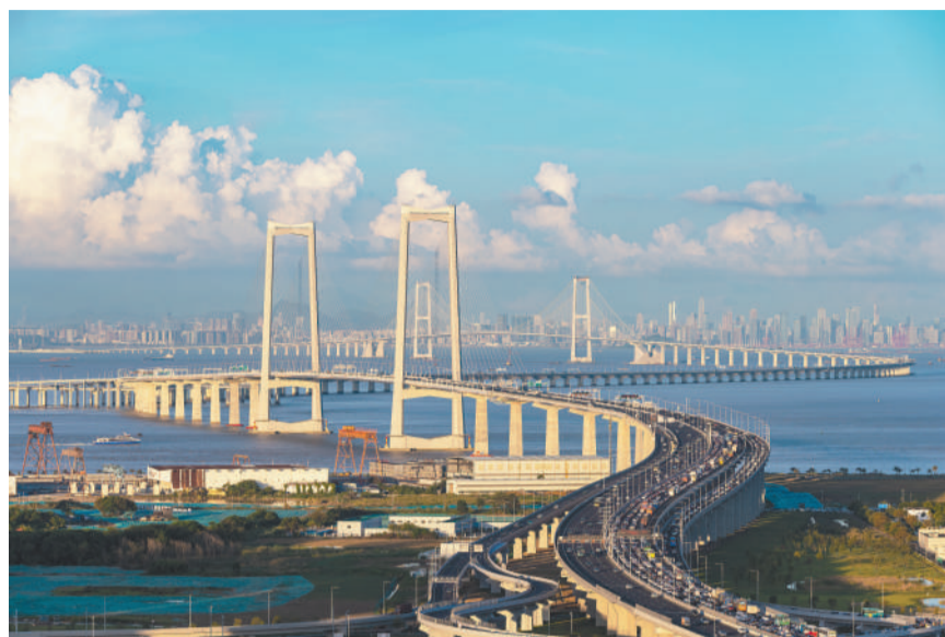
The Shenzhen-Zhongshan Link, opened to traffic on June 30, is a mega cross-sea passage in south China that features two bridges, two artificial islands, and an underwater tunnel. (PHOTO: VCG)
