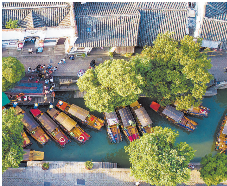
An aerial view of the Tongli Ancient Town in Suzhou, Jiangsu province. (PHOTO: VCG)
