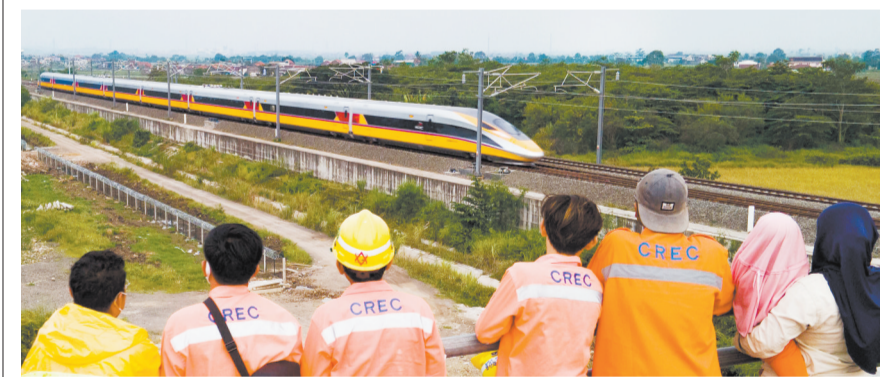
A hot-running test is carried out on a section of the Jakarta-Bandung High-Speed Railway in Bandung, Indonesia. Built with Chinese technology, it is a flagship project that combines the China-proposed Belt and Road Initiative with Indonesia's Global Maritime Fulcrum strategy. (PHOTO: XINHUA)
