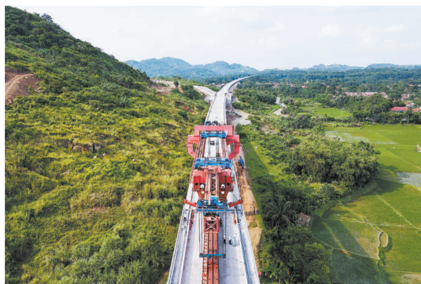
The last box girder along the Jakarta-Bandung High-Speed Railway (HSR) has been erected, laying a solid foundation for the completion of the HSR and its opening to traffic in June 2023. (PHOTO: XINHUA)
