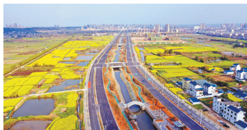
The water diversion project in Taihe county, Jiangxi province, improves the local ecological environment and makes the county more livable. (PHOTO: VCG)
